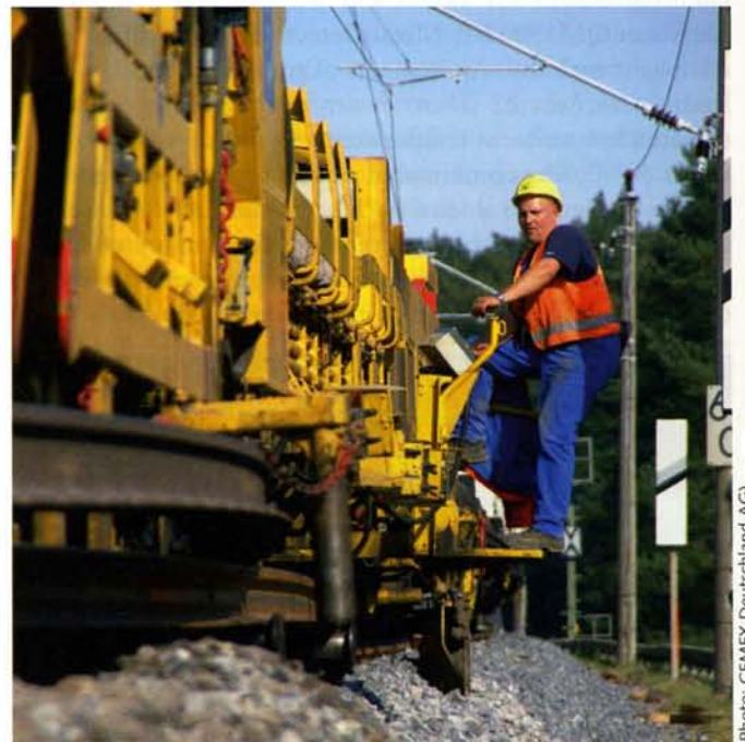
3 The track laying machine renews 150 m of track per hour
